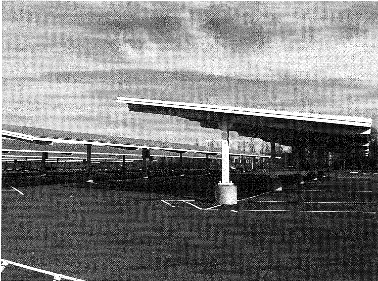
Figure 4. Illustrative Example of Solar PV Carports (from Solano Community College District)
